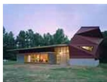
Lucy House-Freear arch. Photo T. Hursley
