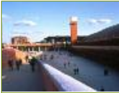
Atocha Station, Madrid, Spain, Rafael Moneo architect, UIA Gold Medal 1996 - Pritzker Prize 1996
