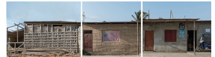
△ Figure 4. (left) Fully exposed elements, untreated, and in contact with the ground. Lifespan: six months to four years. (middle) Lifted off the ground and treated with boron salt for termite protection. Lifespan: up to fifteen years. (right) Protected from sun and water and treated with boron salt. Lifespan: thirty years or more.
