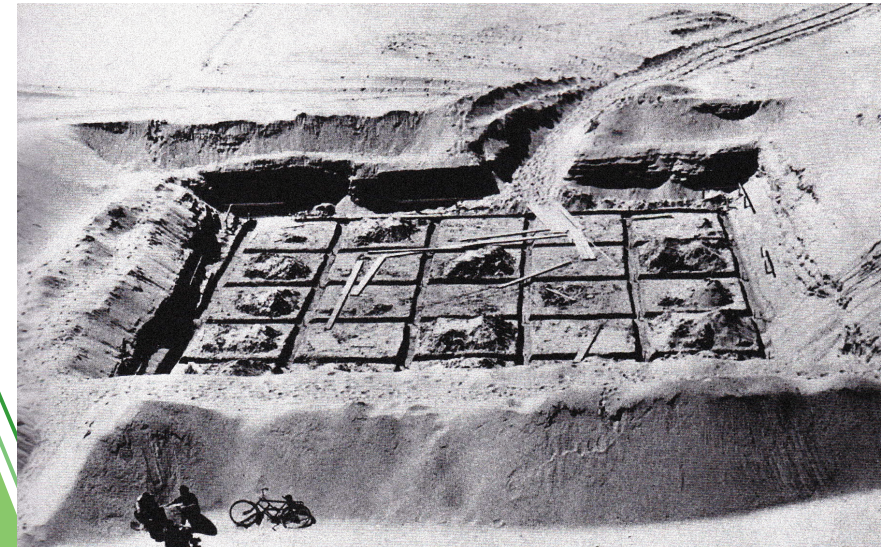
Filling the terrain with sand (draining of the swamp), New Belgrade, 1950's
