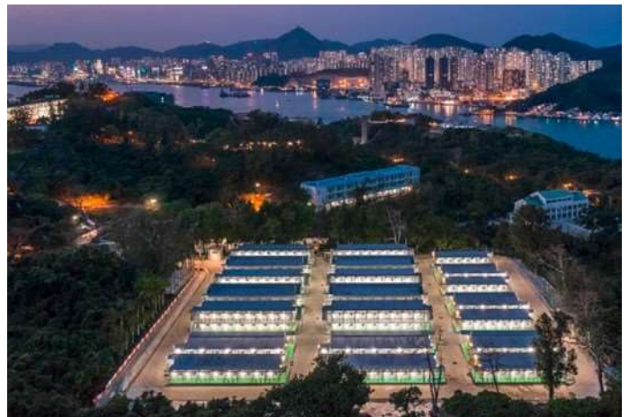
Figure 26. Lower Lei Yue Mun Park – Football Pitch, with 234 units in partially single storey and partially 2 storey high, completed in April 2020 in 56 days
