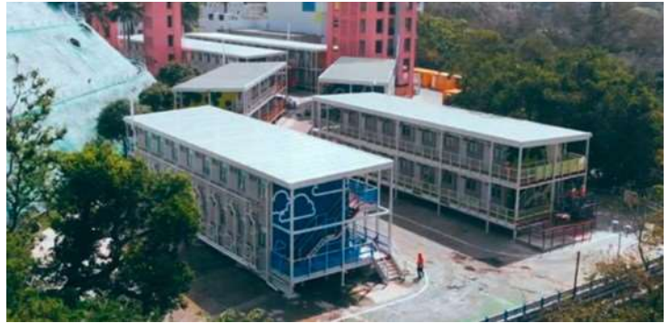
Figure 28. Pat Heung Junior Police Call Permanent Activity Centre, with 120 units in 2 storey high, completed in April 2020 in 66 days.
