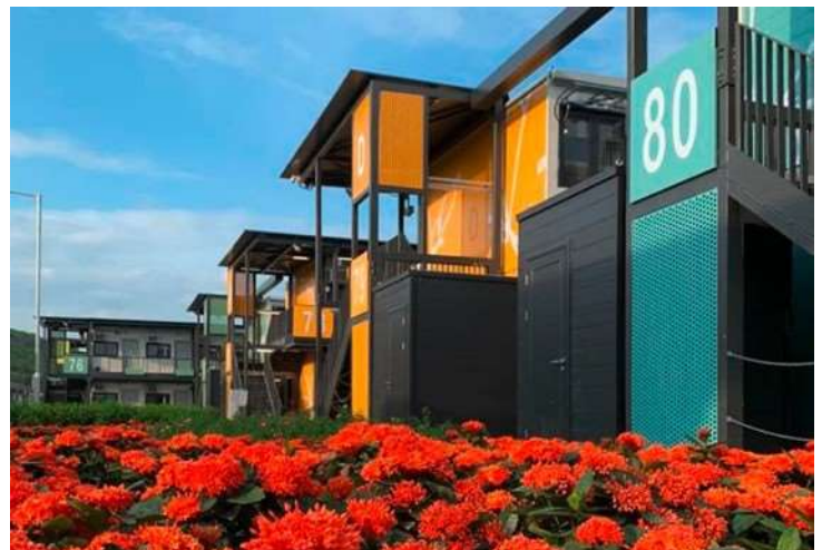
Figure 30. Penny's Bay Phase 2, with 700 units in 2 storey high, completed in September 2020 in 87 days.
