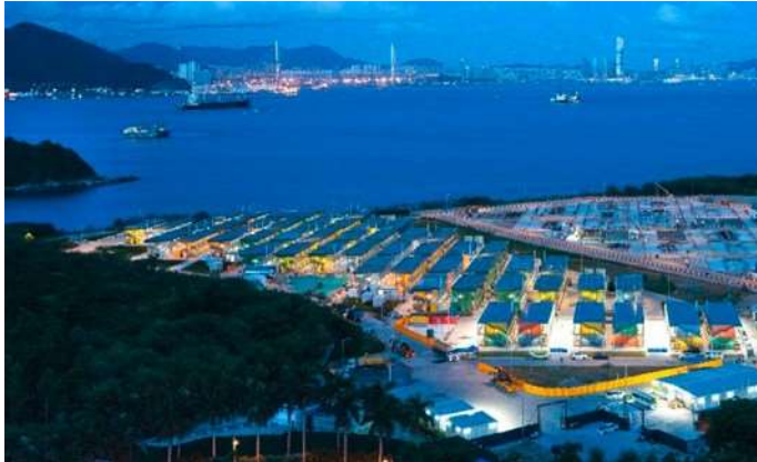
Figure 29. Penny's Bay Phase 1, with a total of 800 units, completed in July 2020 in 145 days.
