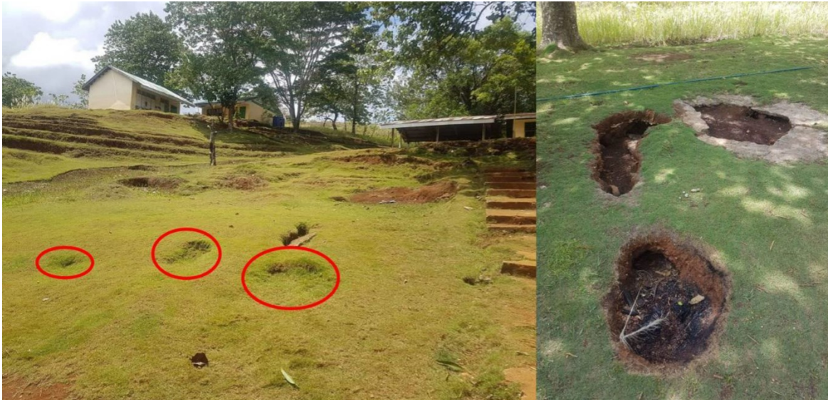
Figure 3. Formations of Sinkholes
